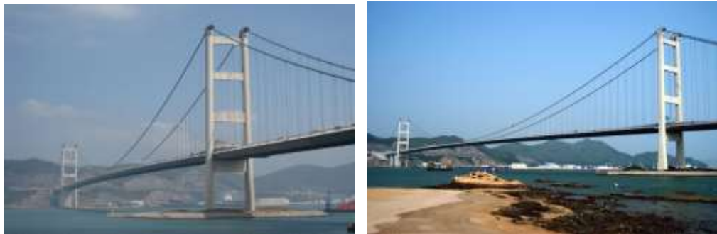
Foto 1 Tsing Ma Bridge : http://www.patnotebook.com/tsing-ma-bridge-photos-and-how-to-get
