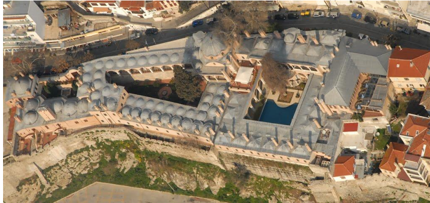
Fig 9. Areal view of the Imaret complex today (source:www.greece.com)
