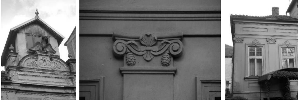
Figure 28, 29, 30: New façade details that decorated new buildings. (Source: K. Elezi)
