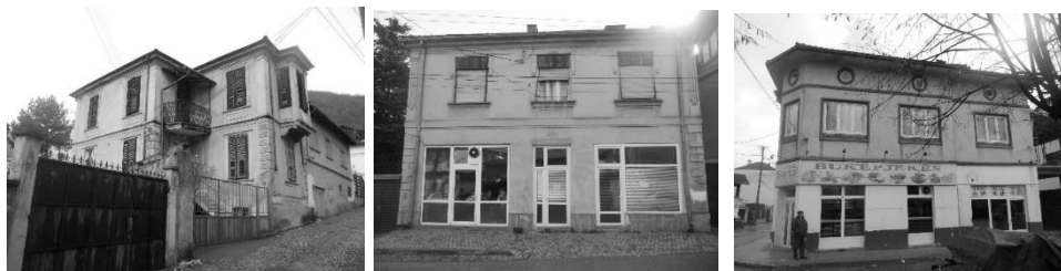
Figure 4, 5, 6: The new buildings were required to look different from what was known as a building “tradition”. (Source: K. Elezi)
