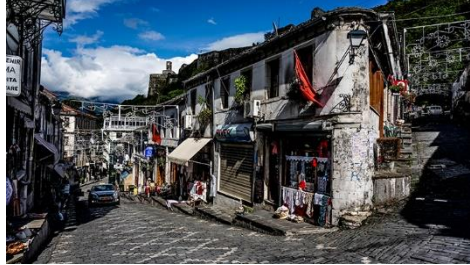
Fig. 8. The main road of the bazaar in Gjirokastra two to three storey buildings and modernized shop fronts.
