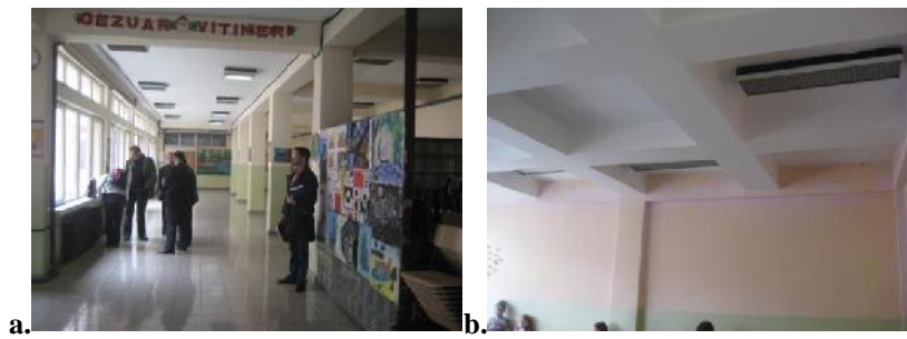
Fig. 1 View of the interior of the school building: a. mainly with windows wrapping and b. mid-floor roof from reinforced concrete
