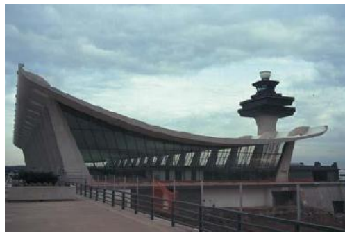
Fig. 2.9 Dulles International Airport, Washington, DC, USA, Saarinen (Eero) and Associates, 1962. Inclined piers support the catenary slab.
