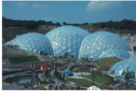
Fig. 2.4 Eden Project, Cornwall, England, Nicholas Grimshaw & Partners, 2001. A cluster of interlinked biomes .
