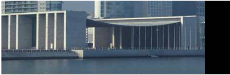
Fig. 2.8 Portuguese Pavilion, Lisbon, Portugal, Alvaro Siza, 1998. The canopy drapes between two porticoes.
