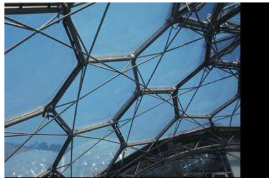
Fig. 2.5 Biome interior structure consisting of outer primary hexagons and an inner layer of braced rods .
