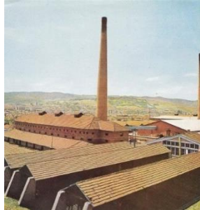
Fig.13 The old state of the factory-outside
