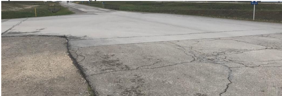
Fig 3: Replaced concrete with asphalt pavement at 1st road intersection on Bondsteel
