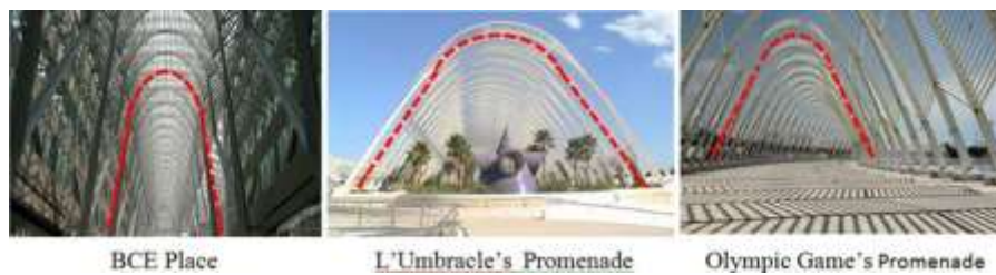
Fig. 11. The steel arches
