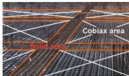
Fig 1 The appearance of cobiax slab surface and the solid area.
