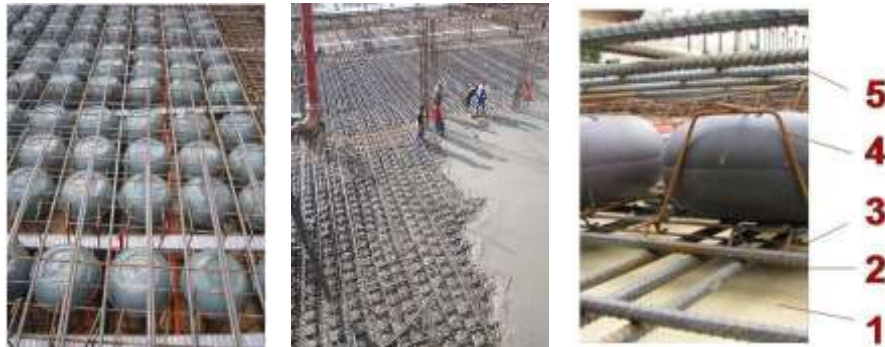
Fig 3 Realization of the slab in workplace
