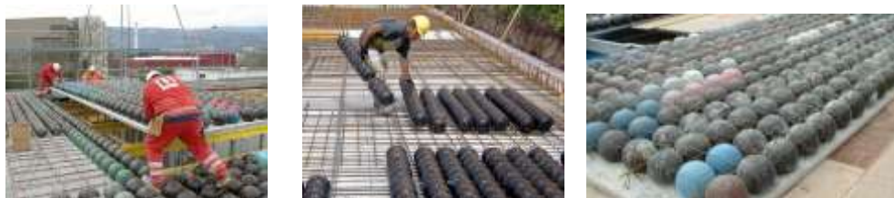
Fig 4 Application of prefabricated slabs in site
