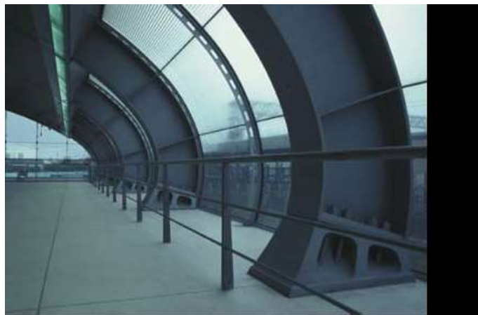
Fig. 5 Curved frames spring from cast-steel bases. Stratford Regional Station, London, England, Wilkinson Eyre, 1999.
