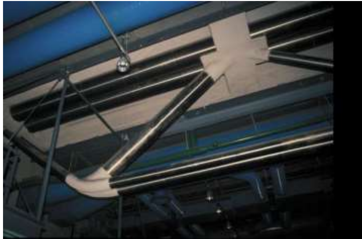
Fig. 4 Double-chords reduce the visual mass of the truss. Centre Pompidou, Paris, France, Piano and Rogers, 1977.
