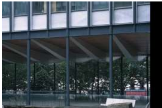
Fig. 3 Beam geometry expresses the bending moment diagram. Jussieu University, Paris, France, Edouart Albert, 1965.
