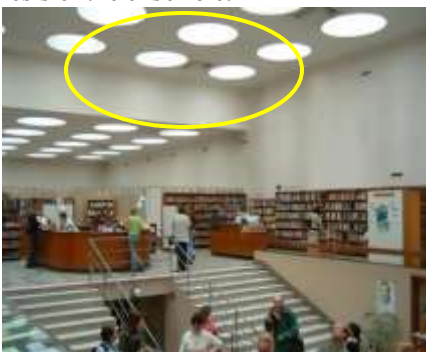
Fig. 27. Interior of conical skylights
