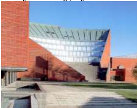
Fig. 24. Image of the building
