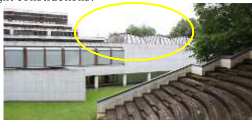
Fig. 3. Elongated skylights of the building
