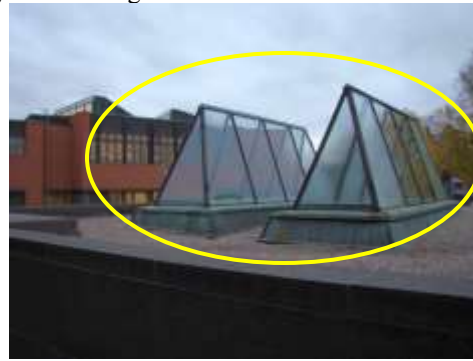
Pic. 25. Image of pyramidal skylights.
