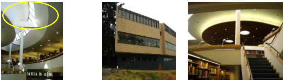
Fig. 10,11, 12. Clerestory skylights and horizontal glazing
