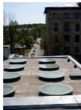
Fig. 28. Exterior of conical skylights
