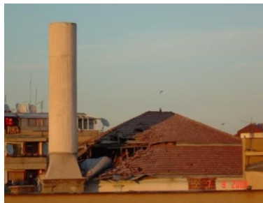
Figure 10 & 11 City Mosque encountered serious structural damage & collapsed minaret over its roof (pictures taken two years after the earthquake incident)
