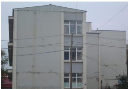
Figure 8 & 9 Non-structural damage of infill walls at high school Arberia, Gjilan
