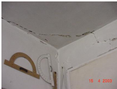
Figure 4 & 5 Typical damage of the school structure Kremenata – Kamenica
