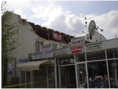
Figure 2 & 3 North side of the Municipal Building with the attic wall fallen down and interior wall damage
