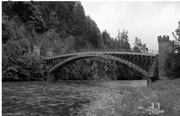
Figure 3.13 Craigellachie bridge, Thomas Telford, Craigellachie, Scotland, 1812 - 1814, l = 50\text{m} [3] - a masterpiece of art.
