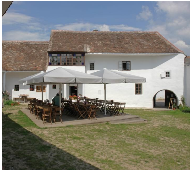
Fig. 2: Brantelhof, Burgenland, Austria. The well maintained earthen building is a landmark in the area. (photo: U. Herbig)
