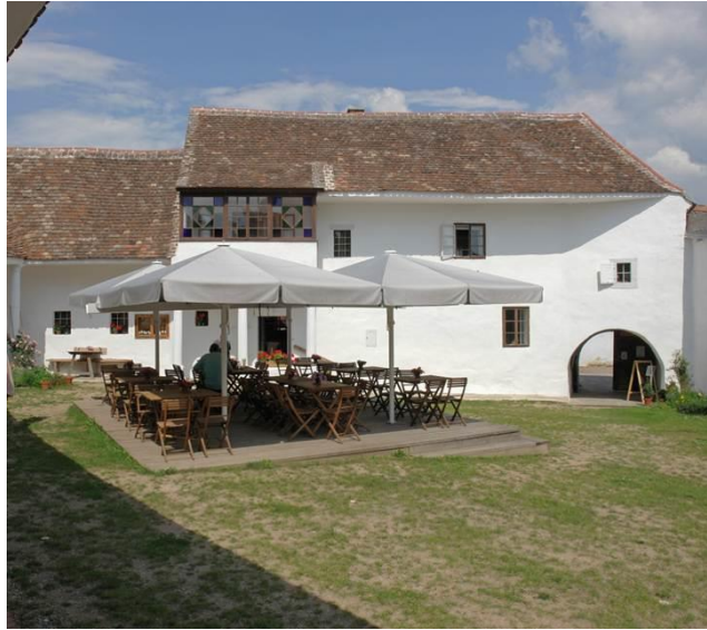
Fig. 2: Brantelhof, Burgenland, Austria. The well maintained earthen building is a landmark in the area. (photo: U. Herbig)
