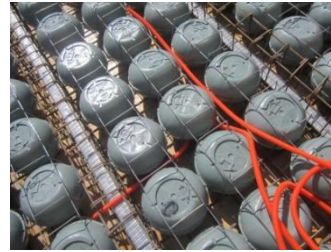
Figure 11. The relieved slab Source; Author's photography in March 2012)
