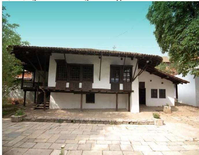
Figure 4 - Example of Banesa with closed qoshk (ground floor+first floor); House of Xhafer Deva built in the 19th Century located in the old core of the city of Mitrovica
