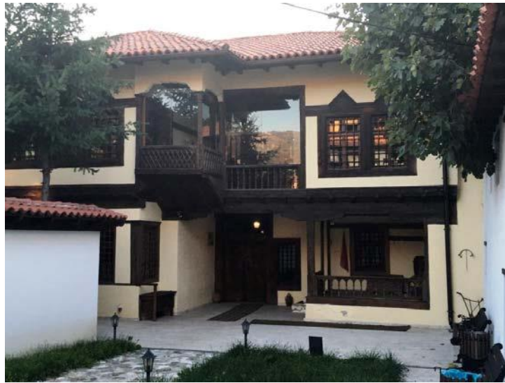
Figure 2 - Example of Banesa with closed çardak. The House of Musa- efendi Sheherzade is located in the plain area of the city, in the "Old Saray" street, built by the end of the 18th century.
