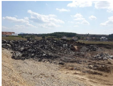
Fig 5. Waste of the removed asphalt layer on the road expanding Skenderaj – Komoran
