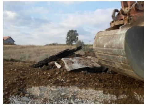
Fig 8. Waste of the removed asphalt layer on the road expanding Skenderaj – Komoran
