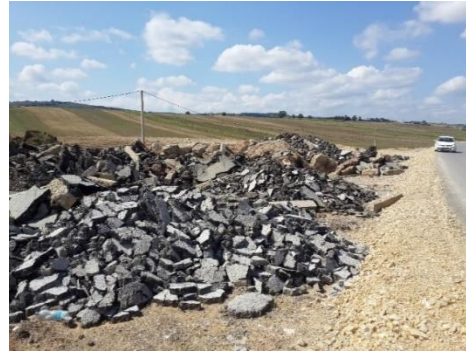
Fig 4. Waste of the removed asphalt layer on the road expanding Skenderaj – Komoran
