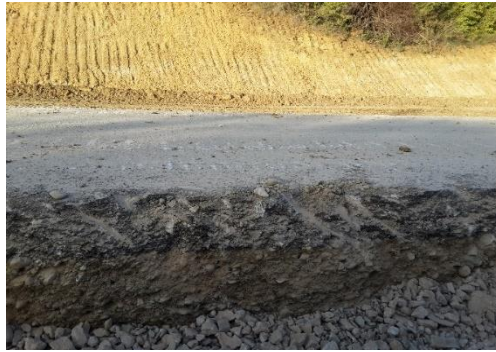
Fig 7. Waste of the removed asphalt layer on the road expanding Skenderaj – Komoran
