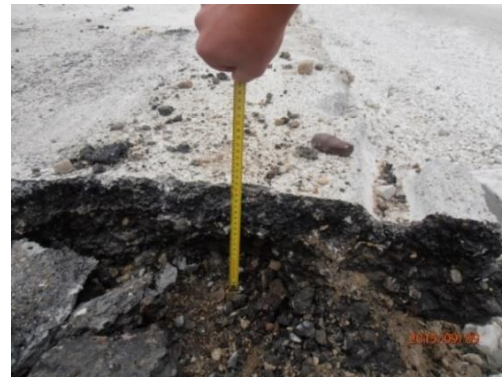
Fig 12. Thickness of the asphalt in place were its starting to remove in the road expanding Skenderaj – Komoran
