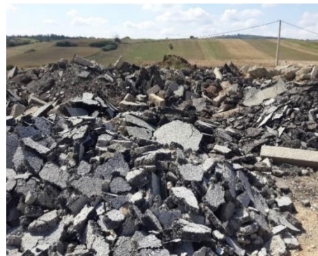
Fig 6. Waste of the removed asphalt layer on the road expanding Skenderaj – Komoran
