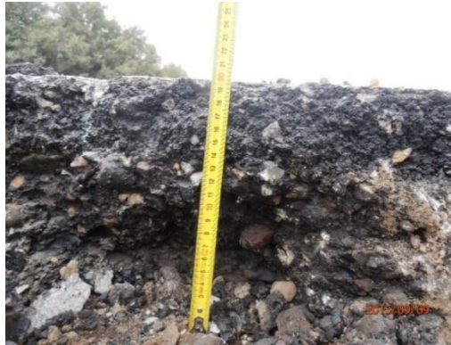
Fig 11. Thickness of the asphalt in place were its starting to remove in the road expanding Skenderaj – Komoran
