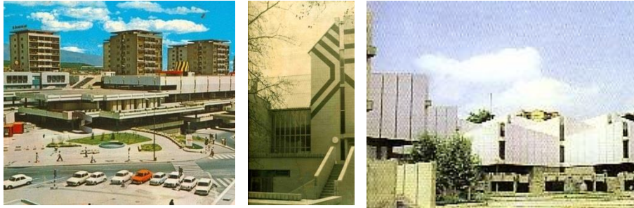
Fig. 25, 26, 27. Ž. Popovski 'City Trade Center' Shkupi, (1973) and 'Pensioners House' Ohri (1973), K. Muratoski and M. Tomić in the 'Ethnographic Museum' (1976) Shkupi. Source: M. Tokarev.
