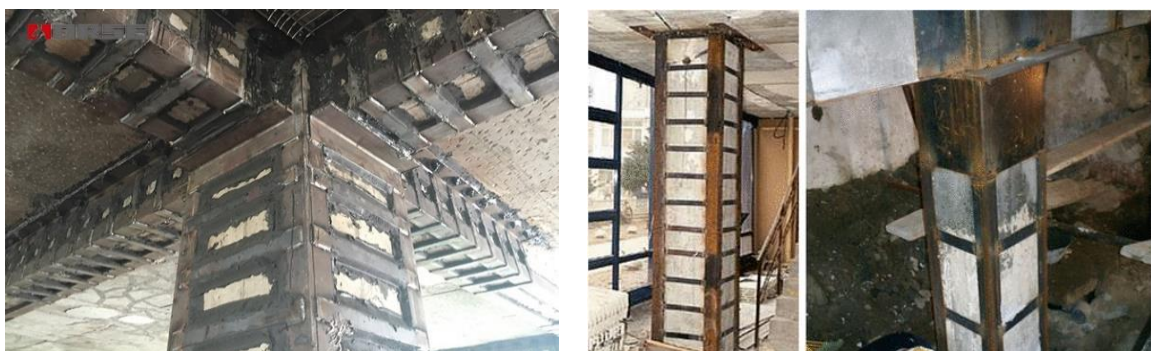
Figure 6. Steel jacketing strengthening method
