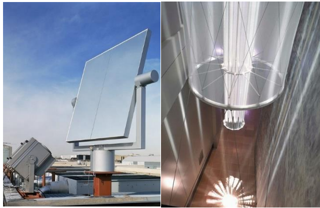
Figure 8 - Forms of lighting in underground spaces ( https://carpenterlowings.com/portfolio_page/solar-light-pipe/ )
