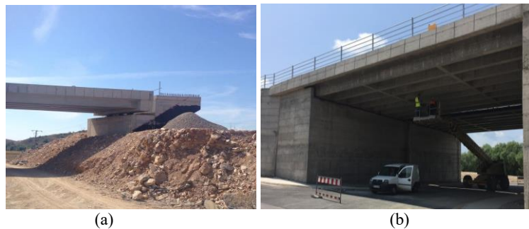
Fig 1. Type of cross section shape used, (a) Overpass on highway Arber Xhaferi R6 type of cross section used is “T” and static scheme is simply supported beam. (b) National road Prishtinë – Pejë type of cross section used is “T” and static scheme is simply supported beam.
