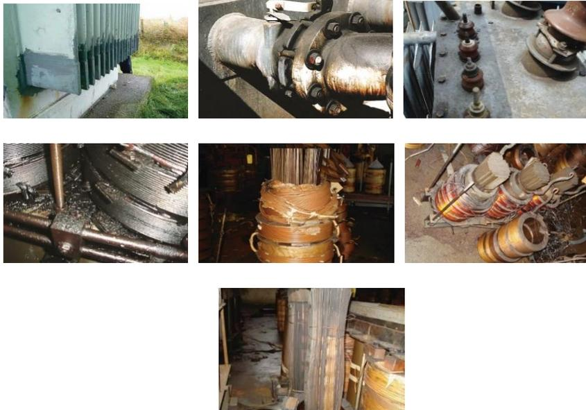
Fig. 3. Failures in the power transformer: (a) Oil leak from the radiator and (b) gaskets; (c) Released connections; (d) Moisture damage to transformer oil; (e) Strengthening the coils; (f) failure due to shrinkage and (g) Failures from magnetic circuit insulation
